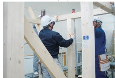
▲ Practical training on building assembly using the wood frame construction method
