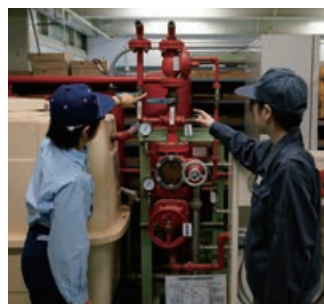
▲ Practical training for comprehensive inspection of indoor fire hydrant equipment (Building Management Technology Department)
